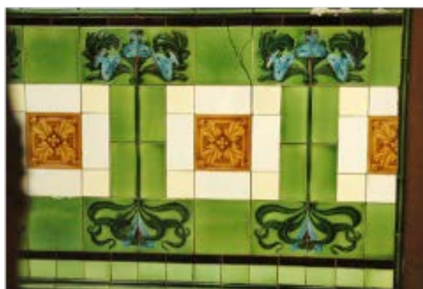
Figure 2 European patterned ceramic tile found on the walls at the ground floor of a double-storey Chinese shophouse in Malacca (Photograph by the author)
