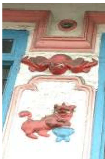
Figure 4 A sculptural plaster or stucco relief of a bat is found on top of another chi lin plaster, or stucco relief on a Chinese shophouse in Taiping, Perak (Photograph by the author)
