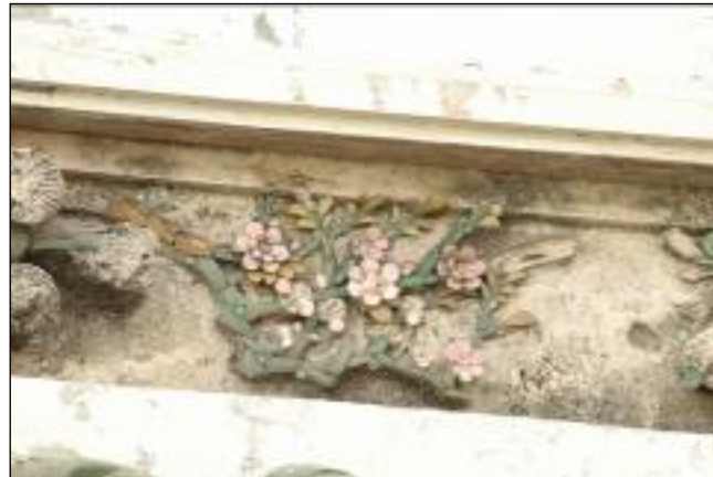
Figure 3 Various shades of colours are depicted on the plastered floral relief which used the ‘ jian nian ’ technique, found on the transom of a double-storey Chinese shophouse in Malacca (Photograph by the author)
