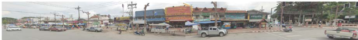
Figure 14 Sight view of street A
