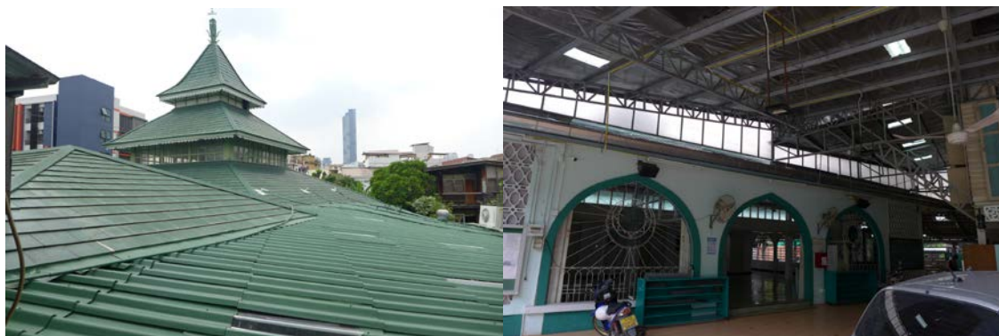
Figure 8 the covered extension in metal sheet
