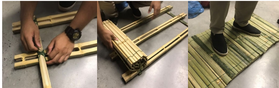
Figure 7 Using rope to hold the structure (left), Laying the floor (middle), and Testing the load (right)
