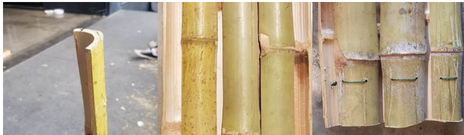
Figure 13 Bamboo cut in half (left), Place the bamboo (middle) and drill a hole for rope upside down (right)
