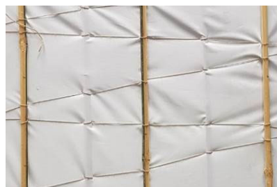
Figure 11 Stretching and tightening the fabric
