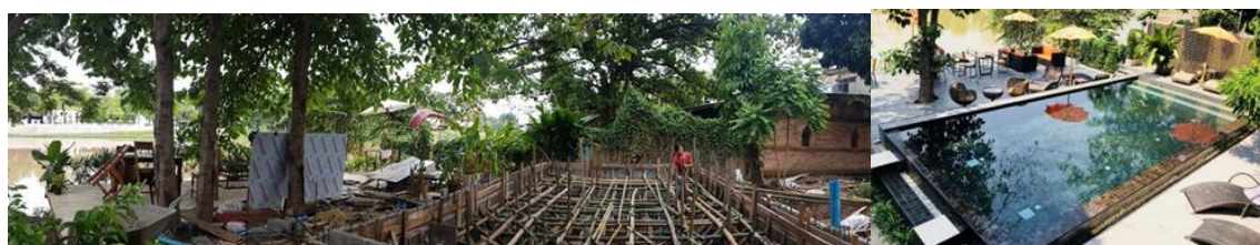
Figure 8 Swimming Pool was placed structural reinforce concrete forms during construction and when completed.
