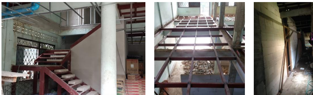
Figure 6 Show pictures during renovation period newly added floor and wall structure were prepared before finishing
