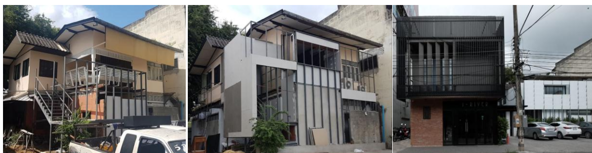
Figure 7 “Villa Section” pictures of being renovated. Adding structure for new stair and panels to wrap old wooden house with a layer of wall was intended to block noise from street and create new face for building (on the right)
